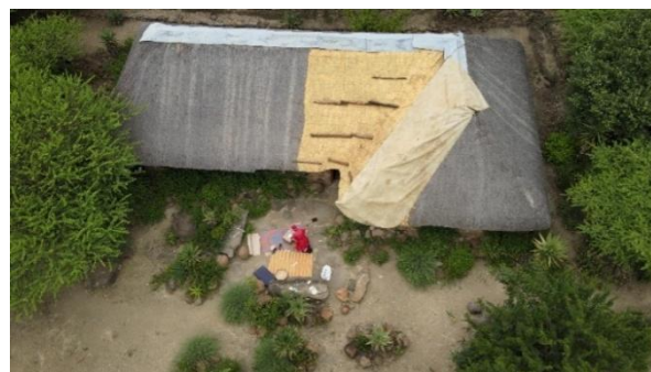
In January work started on partially rethatching the Learning Centre roof to repair the damage caused by old age and termites. A wet summer made it a stop-start operation, but most of the leaks have now been contained.
