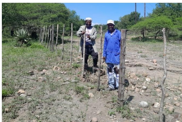
Because fence droppers are highly prized in our valley, theft had made our boundary fence sag when Mandla Magasela and Mondli Mchunu started work on repairs, using Tamboti logs chopped in the bush. The Tamboti tree oozes a poisonous sap which makes the wood difficult to handle and so far our fence has remained intact.
