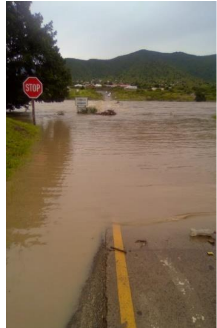
Tugela Bridge at Jacob Zuma crossing
